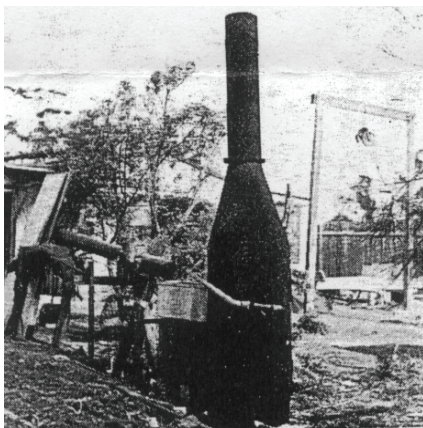
Heath-Robinsonian in appearance, the steam bending plant is in reality efficient and easily manageable.
